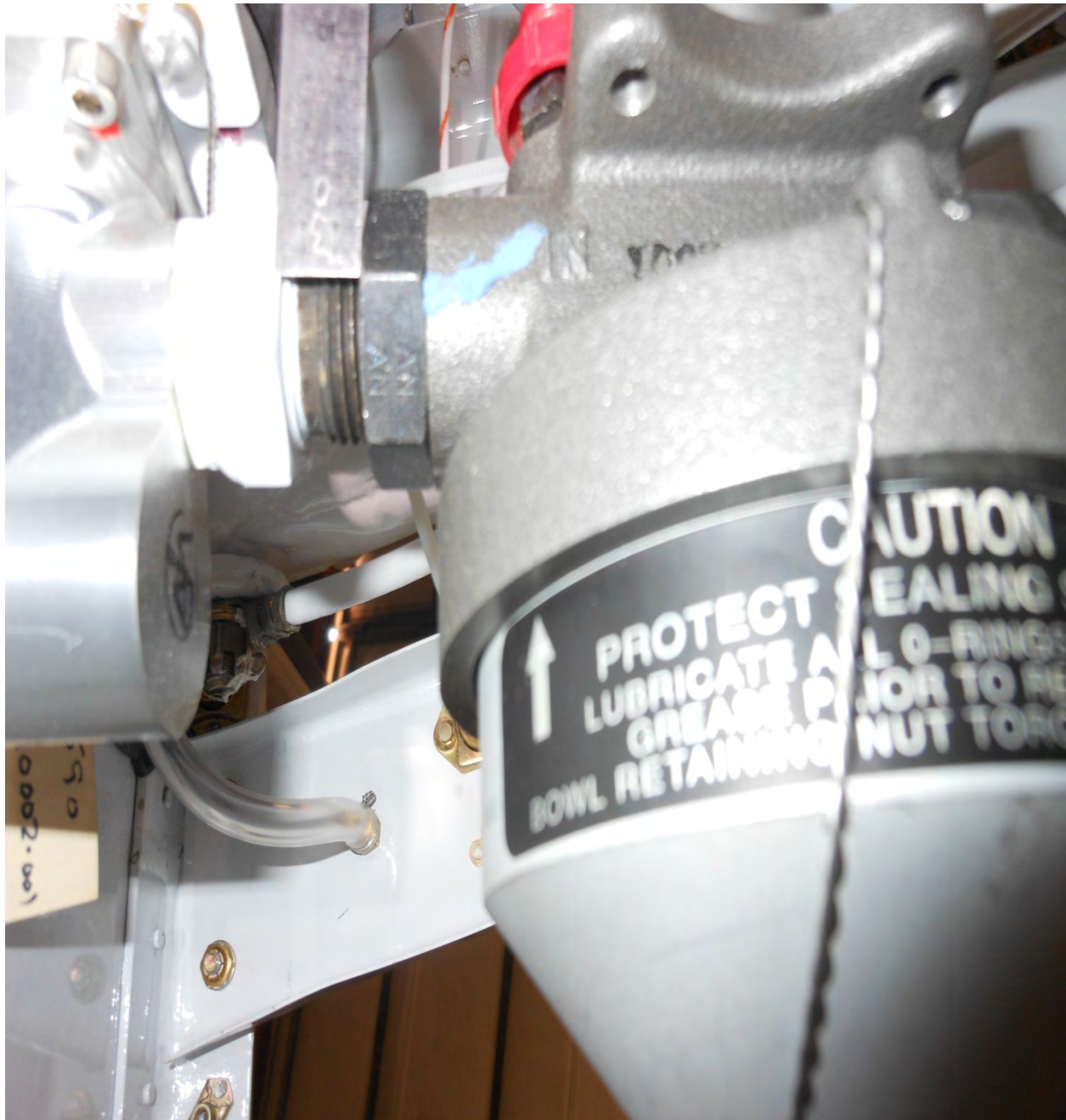
FIGURE 114-4 NON COMPLIANT INSTALLATION
